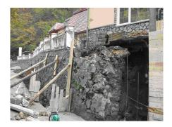
Fig. 16. Temporary blocking the basis and supporting the wall
