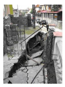
Fig. 6. Formation of massive caverns behind the retaining wall
