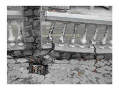
Fig. 4. Degradation of upper wall area and of the protection bulwark
