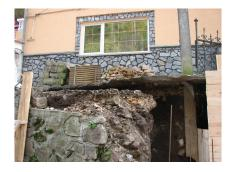
Fig. 5. Break off section of the masonry wall and the crash of the ground behind
