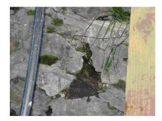
Fig. 8. Wall section with wide cracks, break off of stone masonry and vegetation growth
