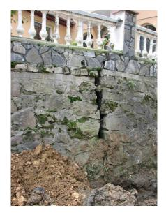
Fig. 3. The large opening of the settlement joint
