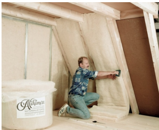
Fig. 10. The manner to mount the layers of mineral wool layers
