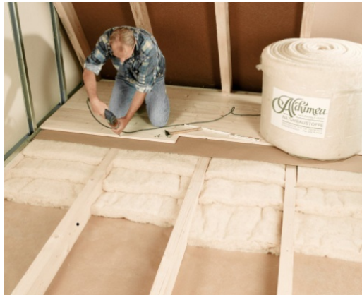
Fig. 11. Method to mount the cellulose fibers insulation
