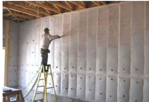
Fig. 11. Method to mount the cellulose fibers insulation
