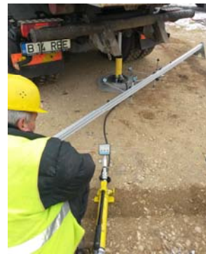
Fig. 2. Plate bearing test
