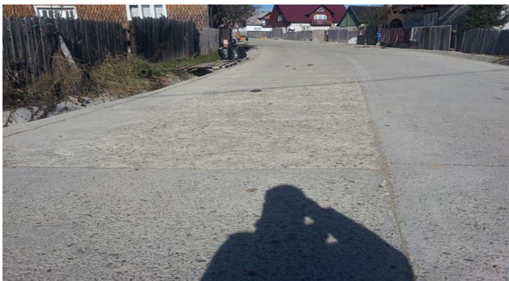
Fig. 3. Exfoliation of the surface
