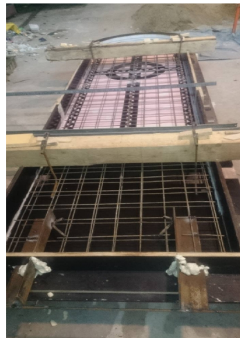
Fig. 8. Moulding the central part of the monument
