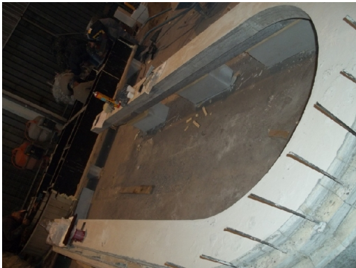
Fig. 9. The resulted self compacting concrete frame
