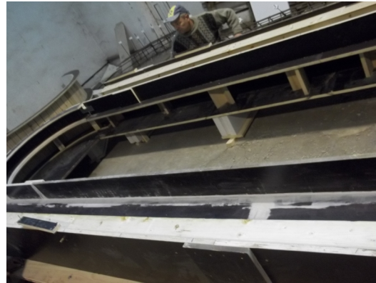
Fig. 3. The wooden cast mould
