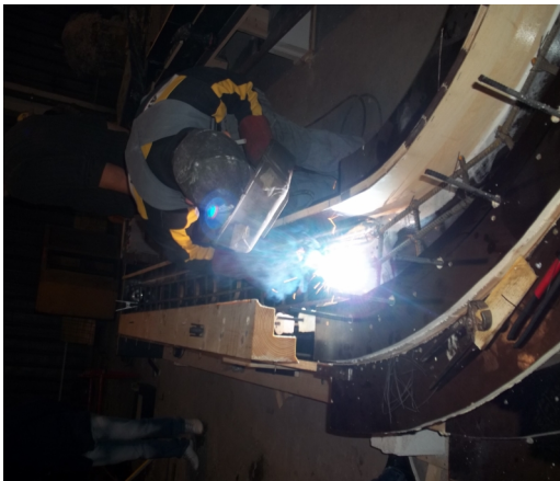
Fig. 6. Welding the rebars
