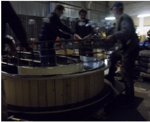
Fig. 5. Placement of the rebars
