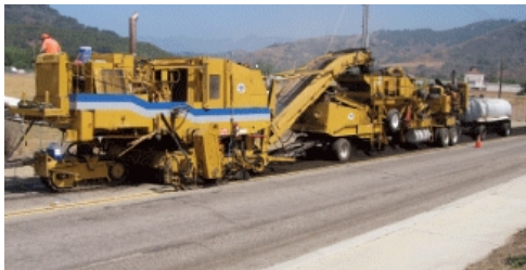
Fig. 5. Cold in-place recycling [10]
