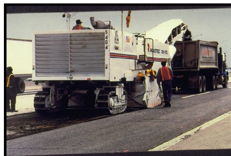
Fig. 2. Hot mix asphalt recycling [1]
