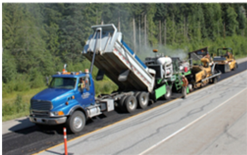
Fig. 4. Hot in-place recycling [9]
