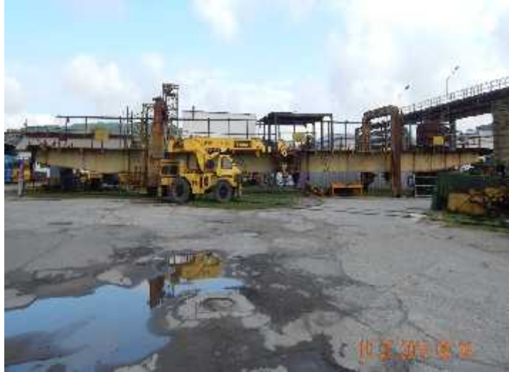
Fig. 9. The disaffected crane
