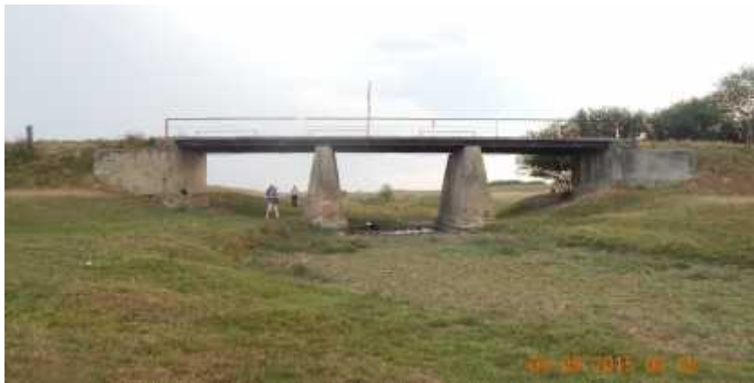
Fig. 2. The existing structure
