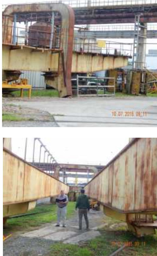
Fig. 10. General view of the crane girders
