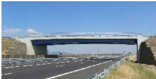
Fig. 6. VFT ® Orştie Overpass on A1 Motorway
