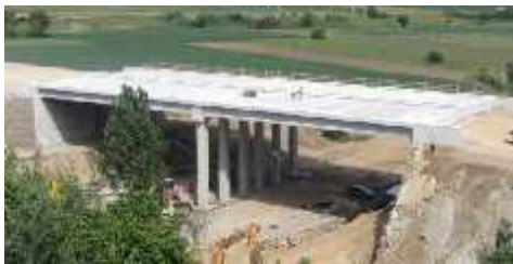
Fig. 3. Executed integral concrete motorway bridges and overpasses
