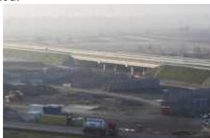
Fig. 4. Motorway viaduct at km 9+405 over the Cugir River (2013)
