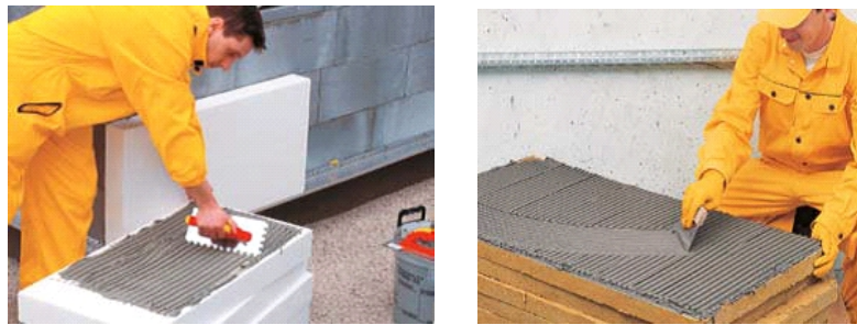
Fig. 7. Proper application of adhesive [5]
