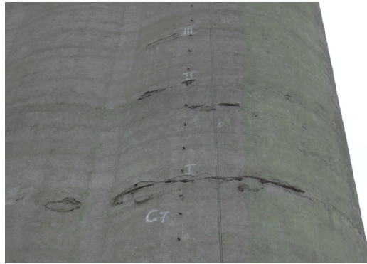
Fig. 3. External cell surface before inspection
