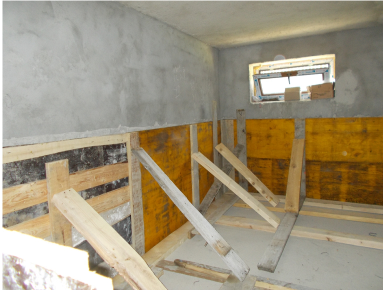
Fig. 7. Execution of inner tank walls
