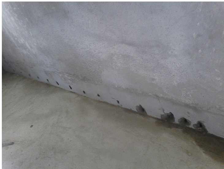
Fig. 6. Waterproofing by injecting Penetron products
