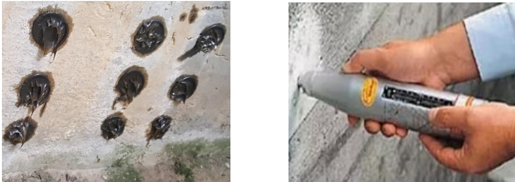
Fig. 12. Sclerometer testing on water tank wall
