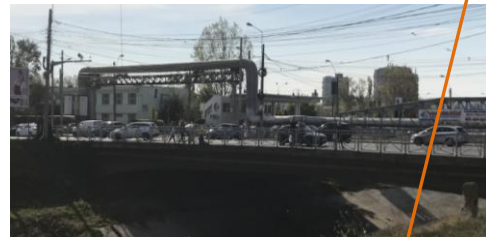
Fig.6 Tudor Vladimirescu Bridge
