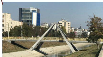
Fig.9. Pedestrian Bridge between Podu Ros and Tudor
