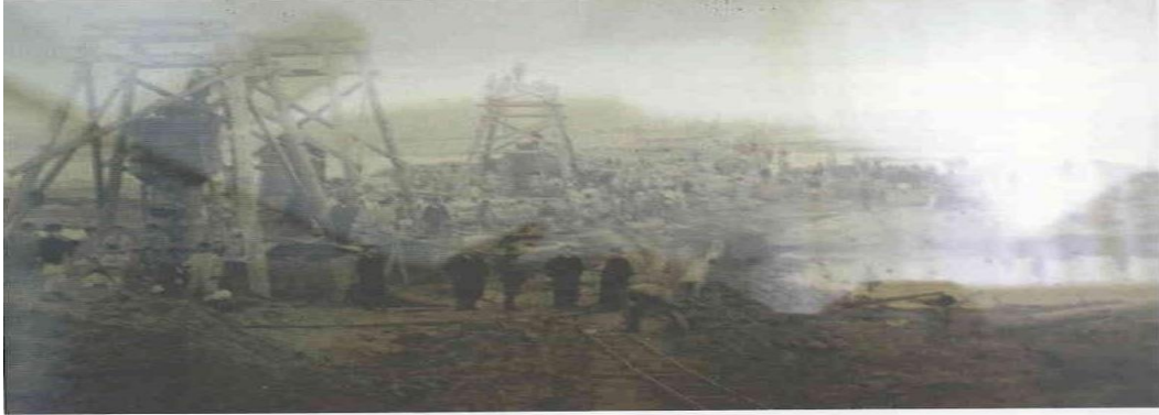
Fig. 1. An image during the execution of the timber bridge. Collection of History Museum of Olt County
