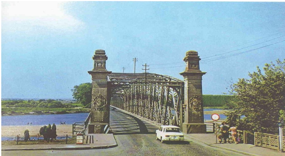
Fig. 4. The bridge entrance portal, modified during communist time. The basket handgrip shaped crossbeam dissappeared
