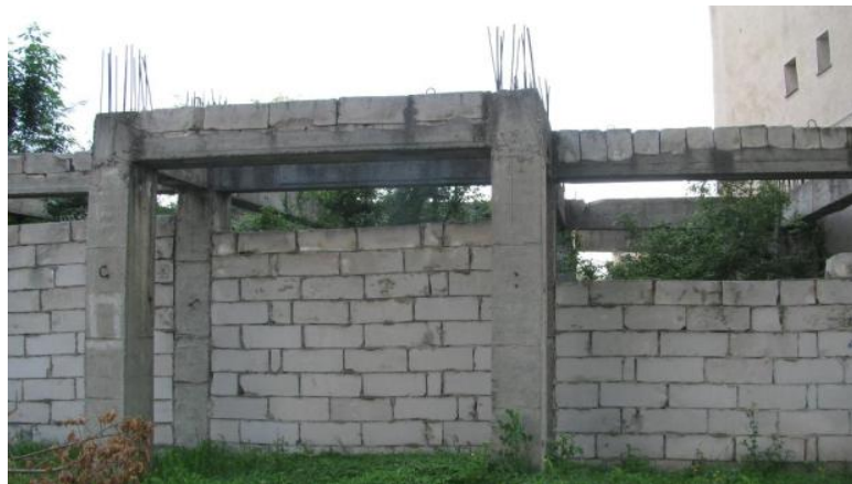
Fig. 1. Actual state of the existing structure
